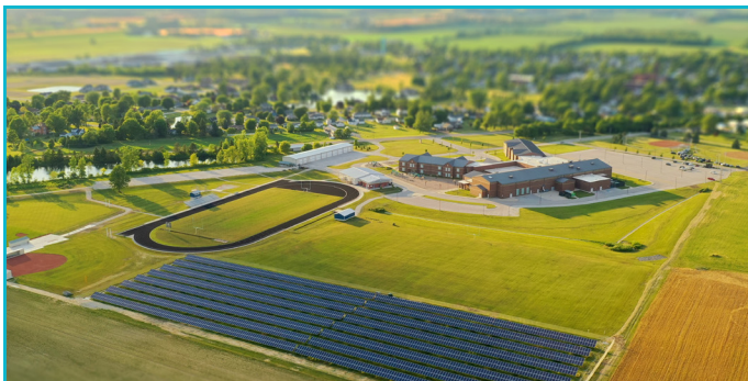
1.1 MW Ohio | Activated in 2020
